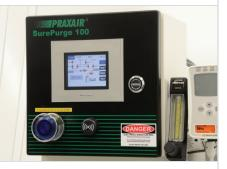
Surepurge 100 PLC Controller Used to control PRS6 Panel Enhanced safety and security through four-level password protocol
