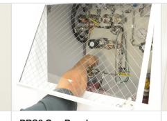
**PRS6 Gas Panel** Removes residual gas and contaminants from the valve connection during cylinder change and maintenance
