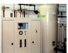
The helium recovery rate for a specialty coatings customer is over 95 percent with a membrane purification system (right).
